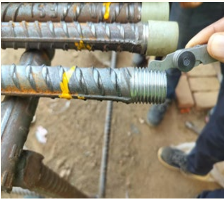
Coupler Thread Checking
