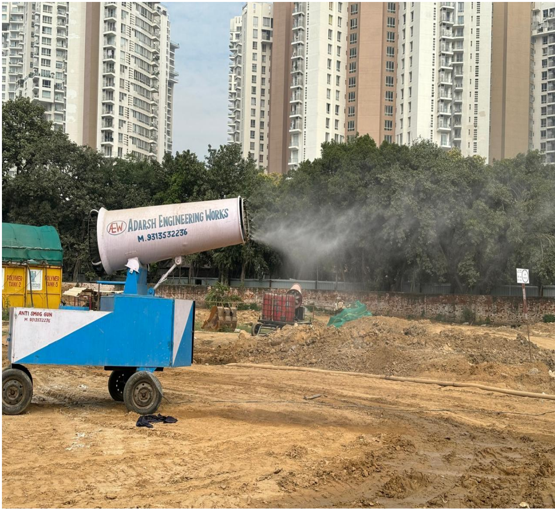
Water sprinkling to control dust spread
