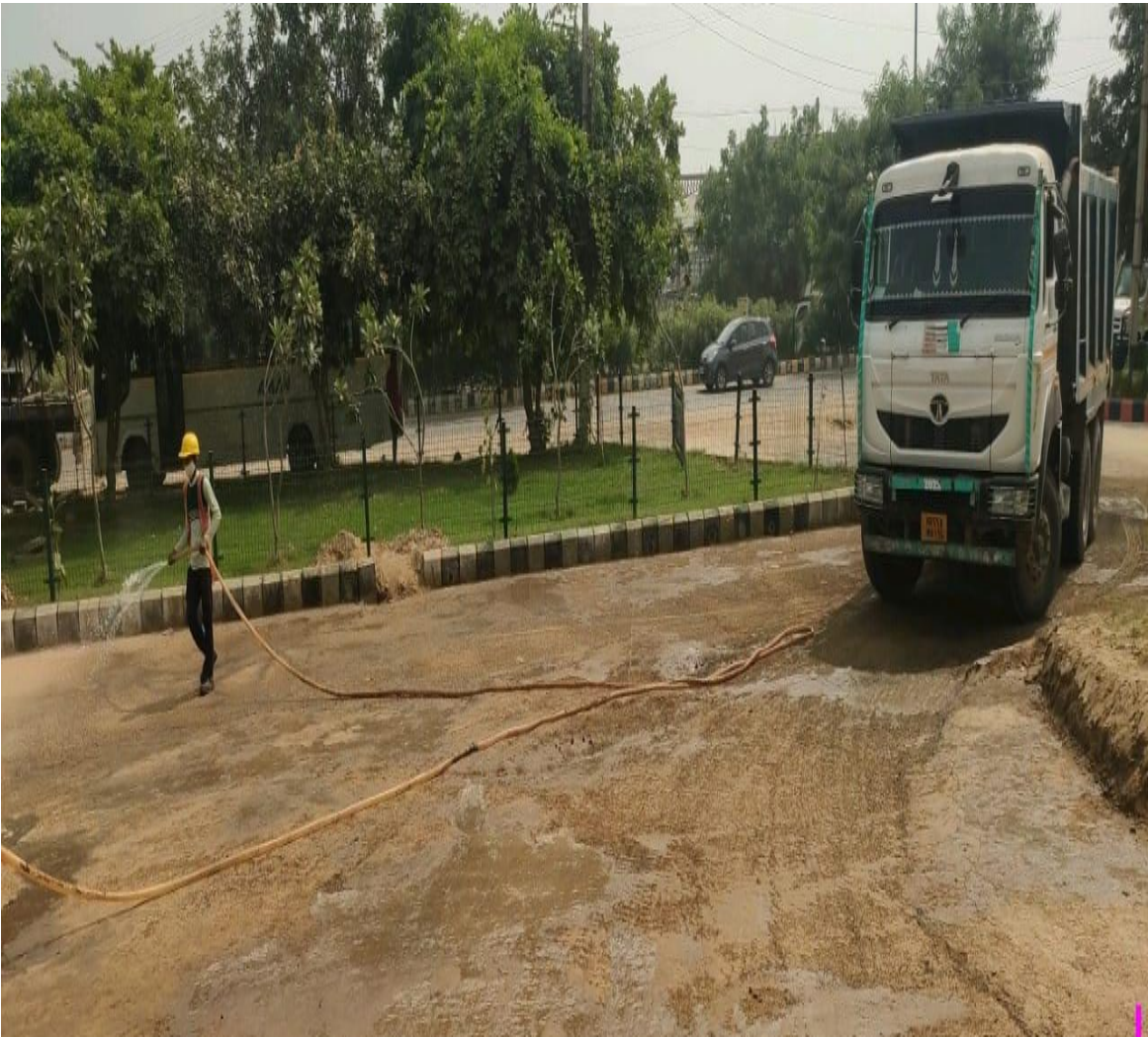
Water sprinkling to control dust spread
